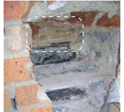
Probe at base flashing reveals moisture bypassing flashing.
