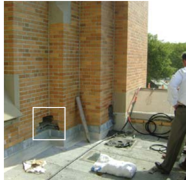
Probe at base flashing reveals moisture bypassing flashing.
