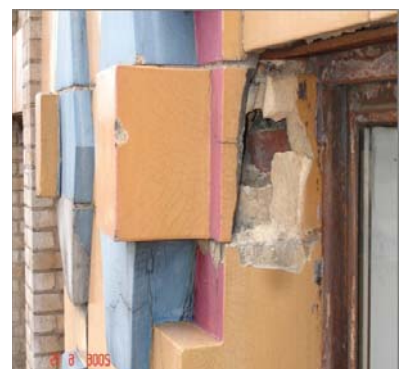
Cracked existing terra cotta; view after removal of loose terra cotta.
